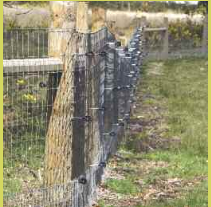
In the summer of 2010 a 900m fence was erected following specification guidance from Natural England. The fence was made of 125 cm high galvanised 'pig netting', with a 'skirt' of buried weld-mesh running horizontally around the inside of the fence to help prevent the beavers digging underneath. Two strands of electric wire were secured around the inside perimeter of the fence, powered with a large battery with a solar panel charger.
