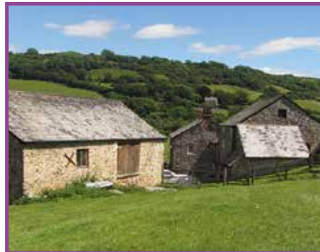
Photo: Branscombe barn
