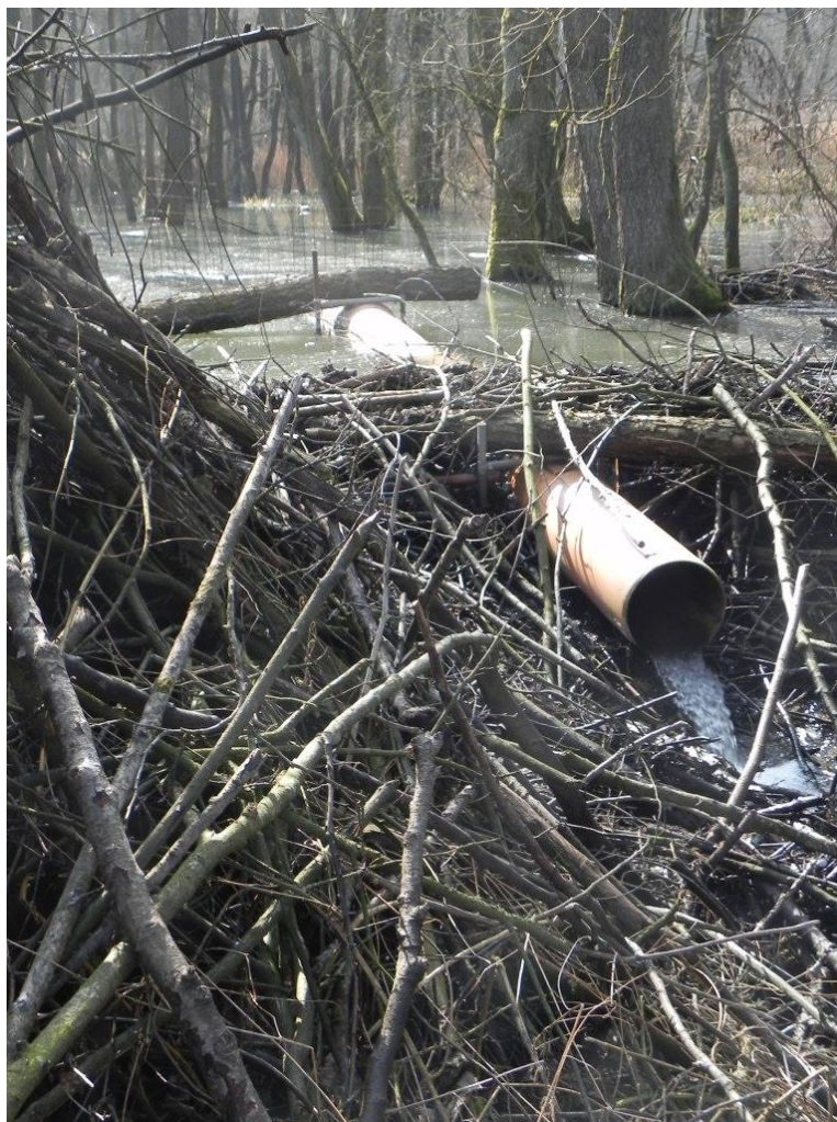
A “Beaver Deceiver” flow device allows the height of the dam and extent of the flooding to be managed without destroying the dam or wetland.
