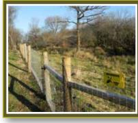
fence has electric strands to prevent beavers climbing and a weldmesh apron on the inside to revent them burrowing underneath. This fencing to construct
